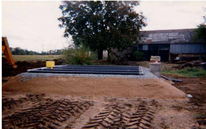
Fig. 4. *TERTRE D'INFILTRATION*
